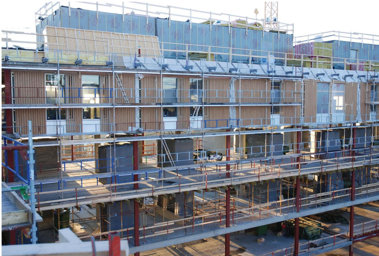
St Olavs Hospital - Industrialized production
